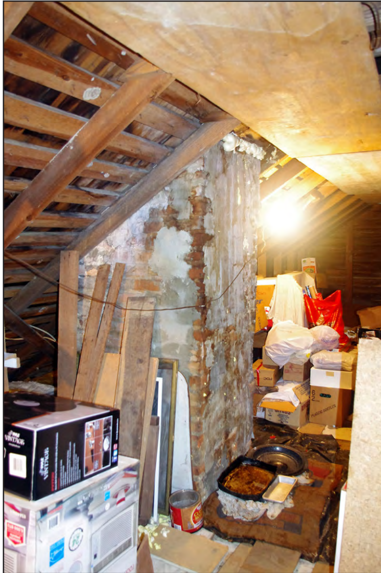
PLATE 41: Interior of Maggie E. Murdoch Watson House, Attic Detail, Looking Southeast
