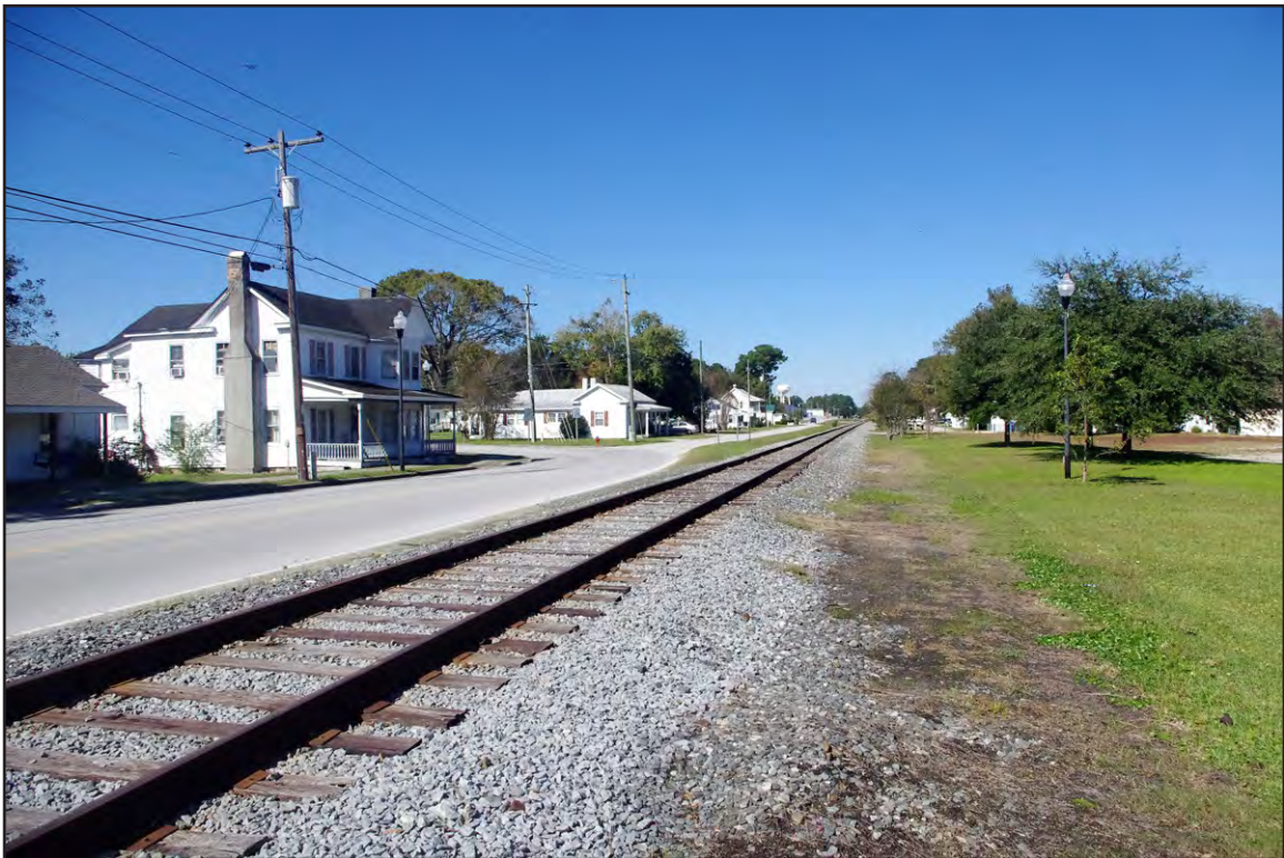
PLATE 58: Newport Historic District (CR 1319), Facing Northwest Toward W. Railroad Boulevard and the Norfolk Southern Railway, Newport, Carteret County
