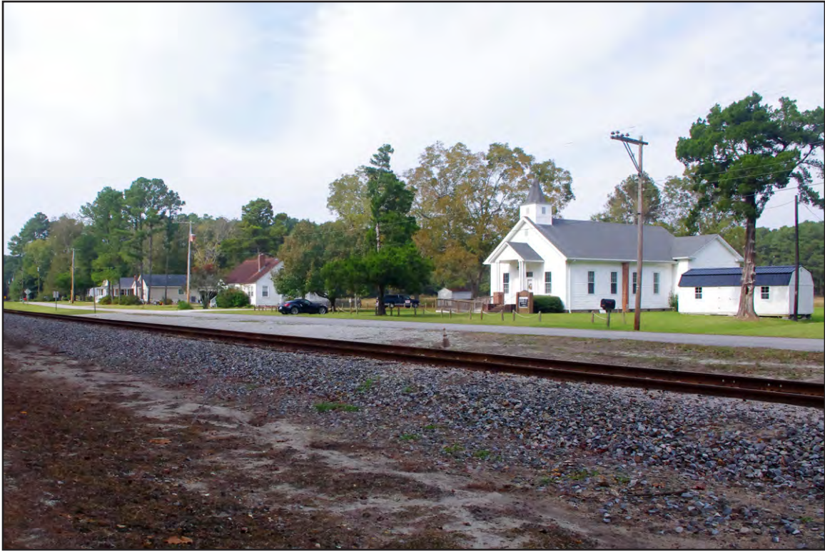
PLATE 65: Norfolk Southern Railway Line and Wildwood Road, Facing Northwest, Wildwood, Carteret County
