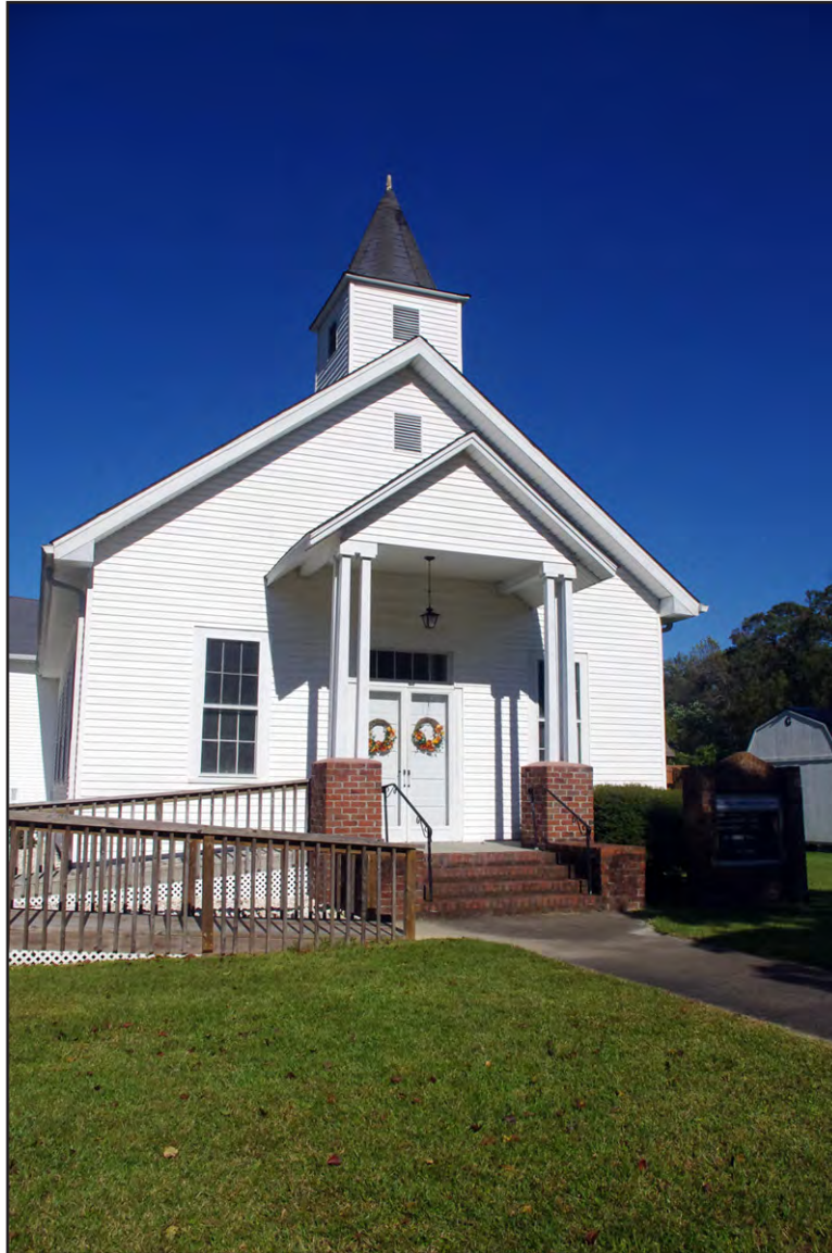
PLATE 5: Wildwood Presbyterian Church, South Elevation, Looking North
