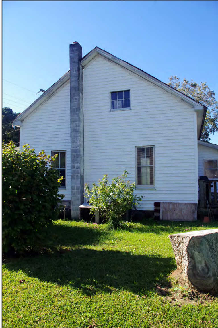
PLATE 22: Albert Clyde Murdoch House, East Elevation, Looking West
