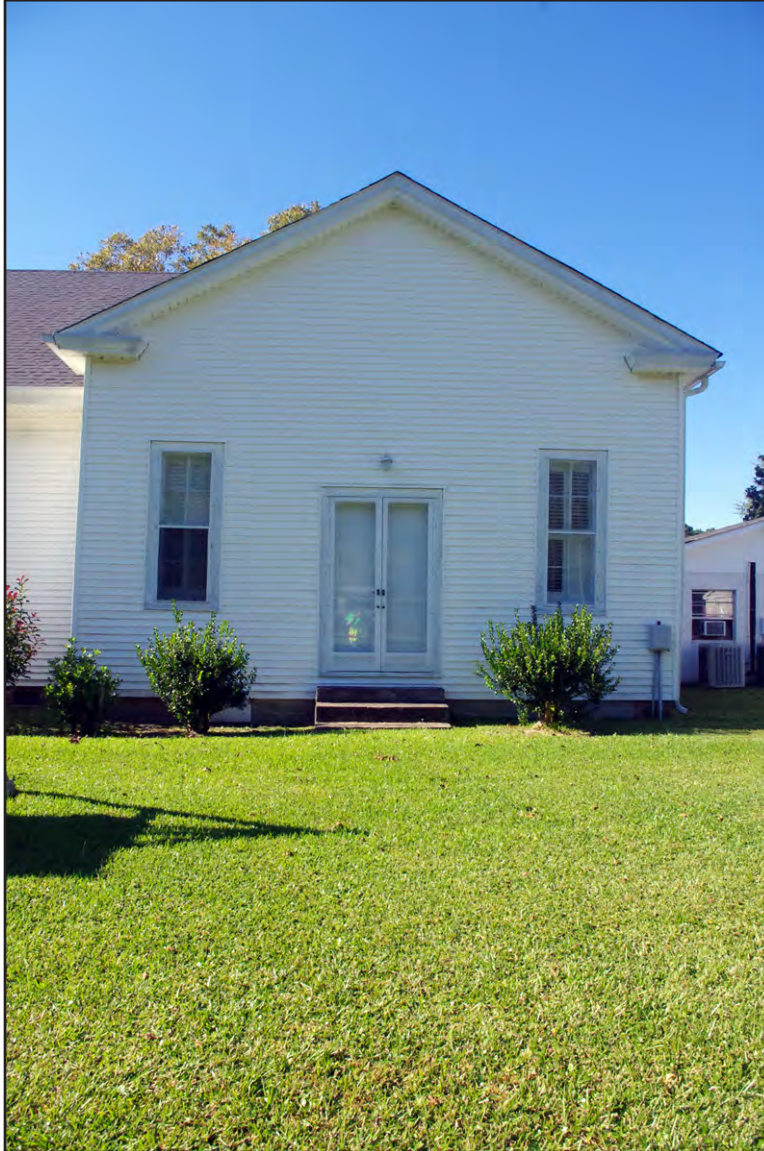
PLATE 7: Wildwood Presbyterian Church, East Elevation of ca. 1893 Wing, Looking West
