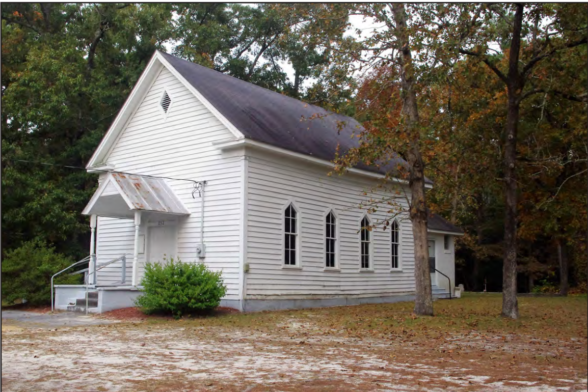
PLATE 17: Peletier Unitarian Church (now Peletier Community Building) (CR1365)
