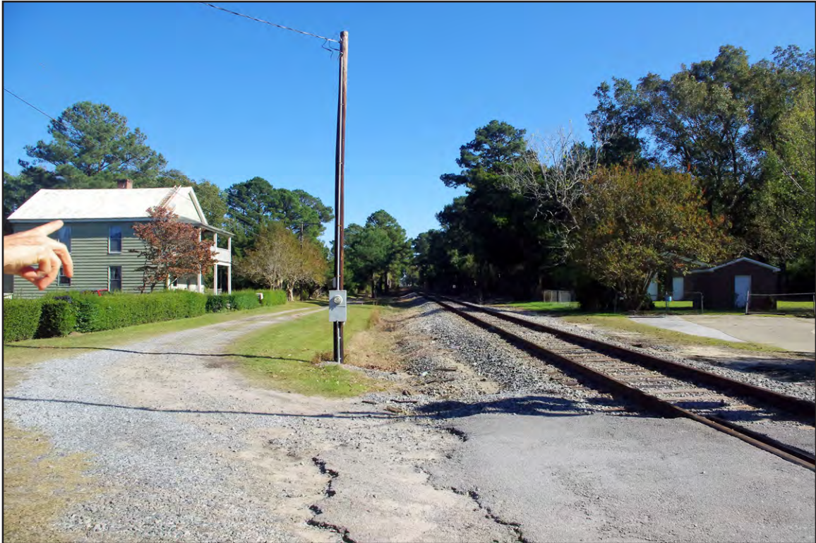
PLATE 30: Wildwood Road at the Intersection of the Norfolk Southern Railway Line, Looking East
