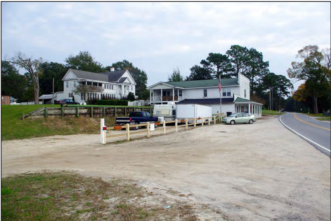
PLATE 56: Stella Historic District (CR0762), Wetherington Landing Road, Looking Northeast
