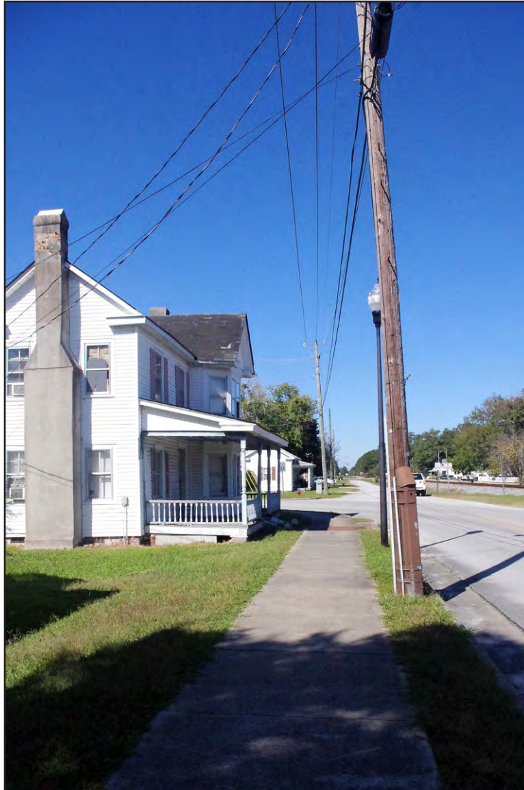
PLATE 46: Cicero Mann House (CR 1297), Oblique View of South and East Elevations
