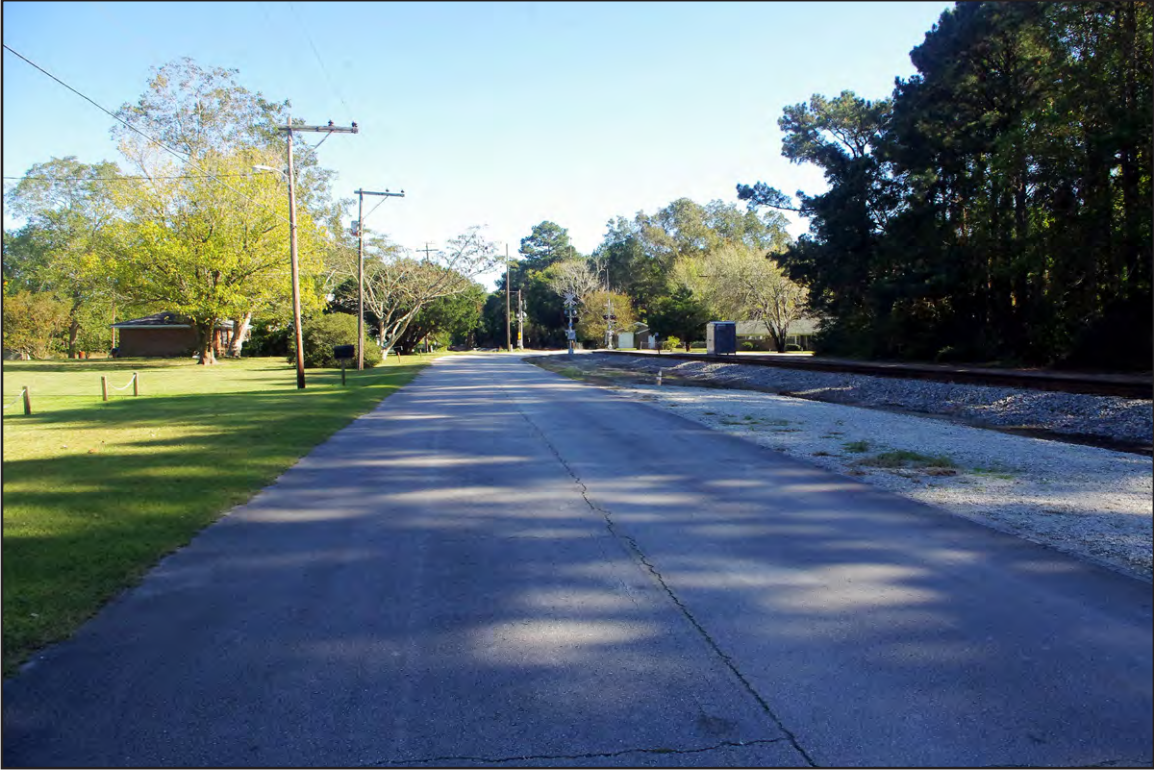
PLATE 50: Norfolk Southern Railway Line and Wildwood Road, Looking East
