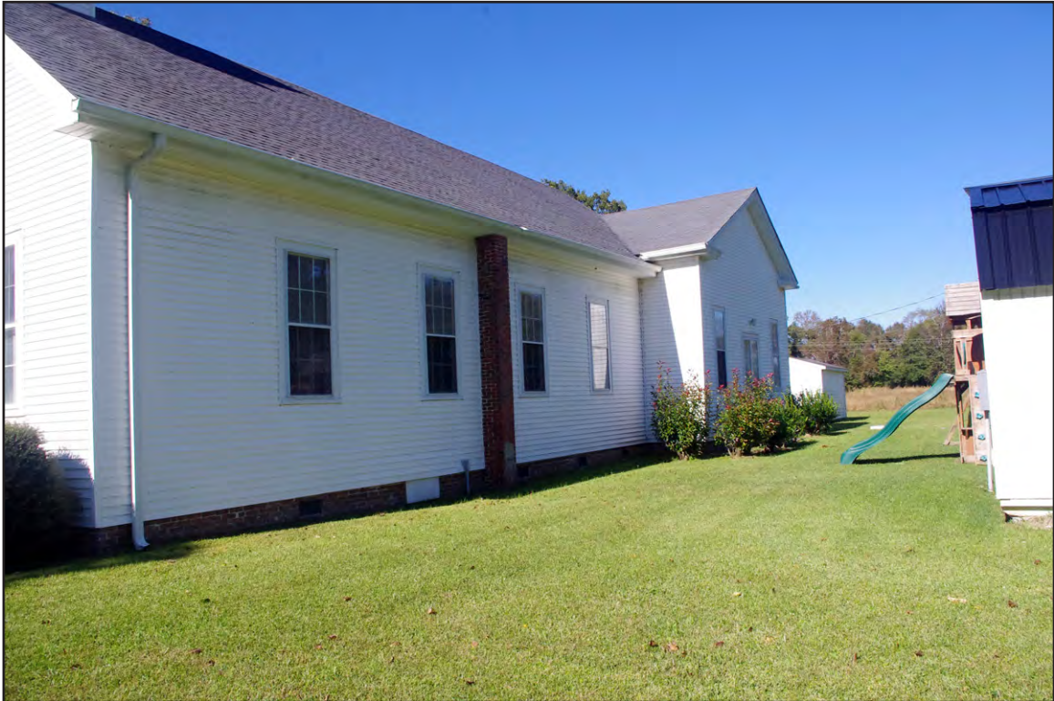
PLATE 6: Wildwood Presbyterian Church, East Elevation, Looking Northwest
